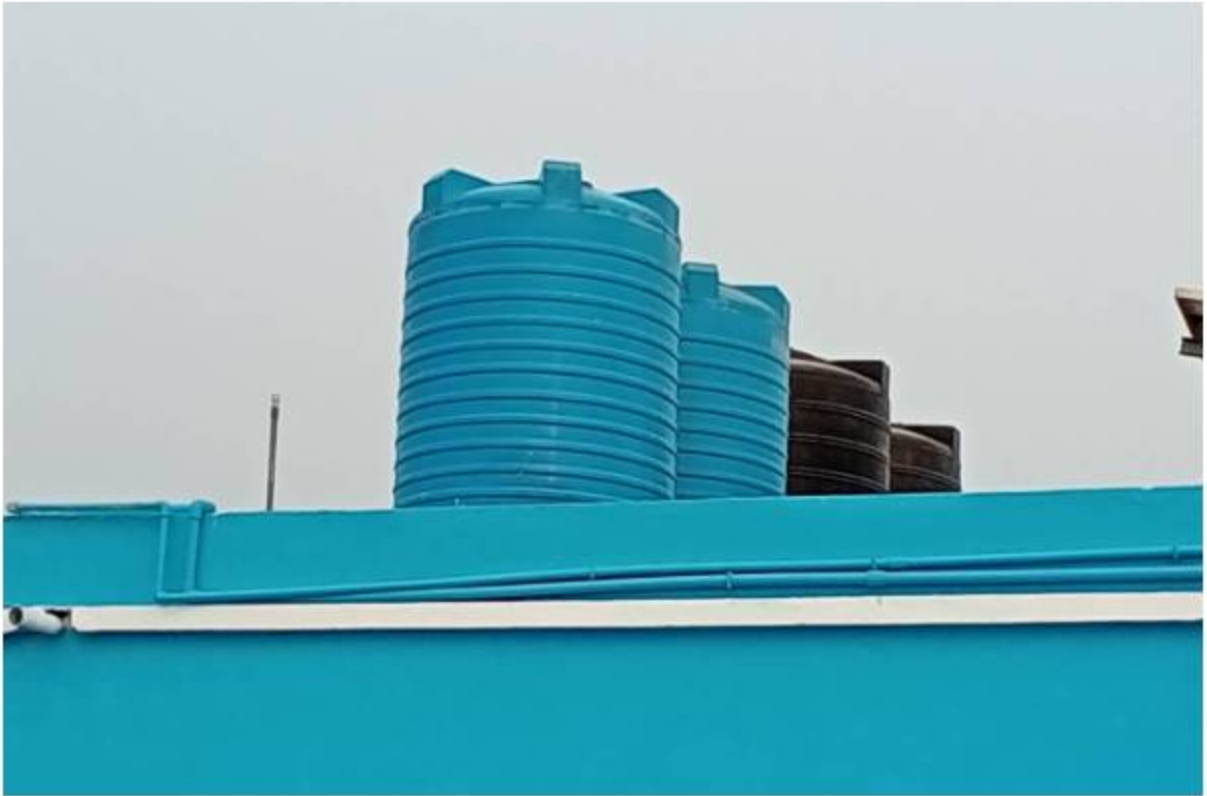
Fig.2: Water Storage Tank
